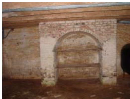
Foundation for the two fireplaces
